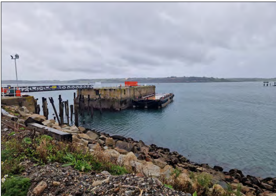
Plate 3) View of the open revetment at the northern end of Northern Arm, facing northeast.
