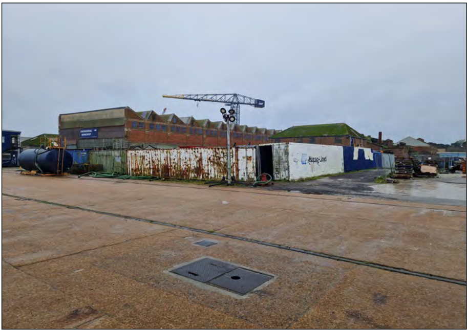
Plate 1) view over the southern section of the Site showing the former 20th century workshop, facing southeast.
