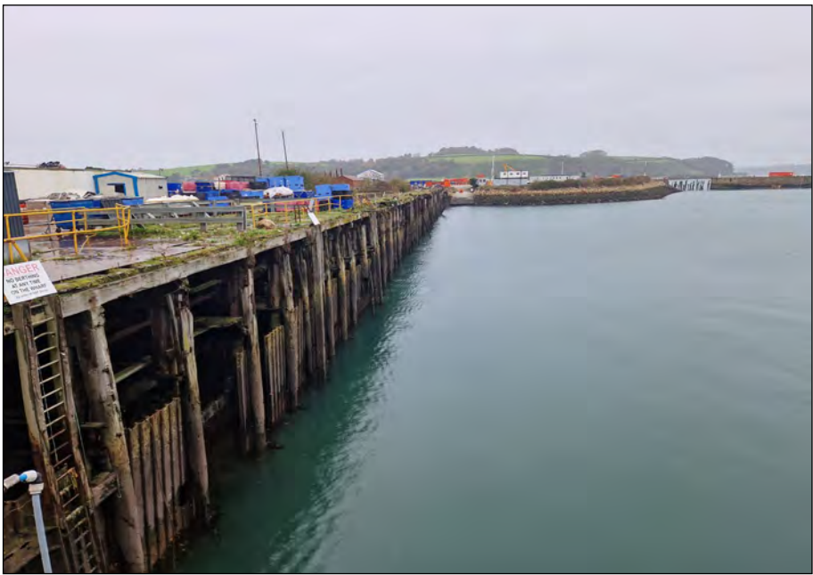
Plate 5) View of the timber structure on the eastern side of the Northern Arm, facing north.
